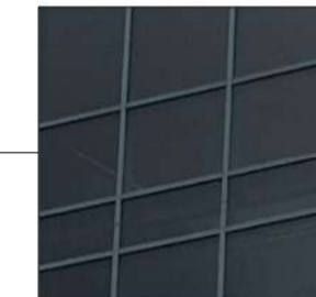
Glazed stair core
