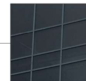
Glazed stair core
